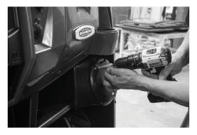
Step 12 - Once secure, make your speaker wire connections and reassemble the top dash panel securing it in place with the hardware removed in previously.
